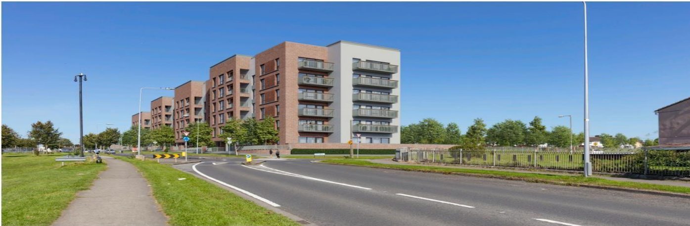
Figure 3: View Looking North
