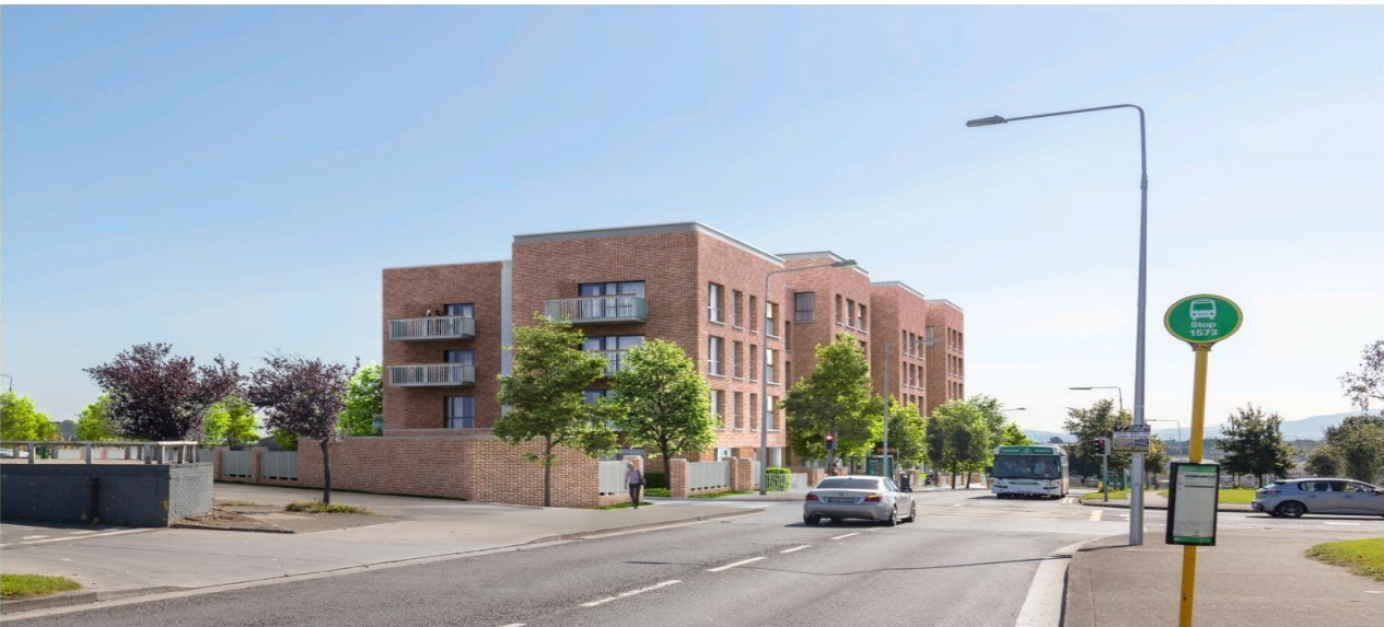
Figure 4: View Looking East along Cardiffsbridge Road
